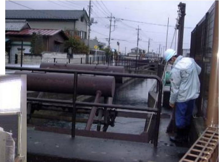
Canal Gate Operation & Patrol
