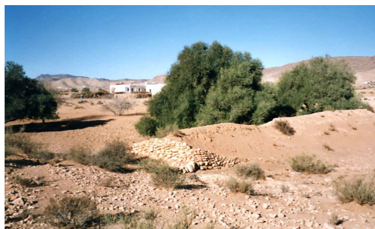
Figure 17: Dam with spillway (Photo: Meinzingner)
