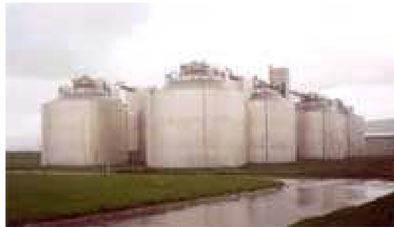
Figure 3: Ankara Sludge Digester
