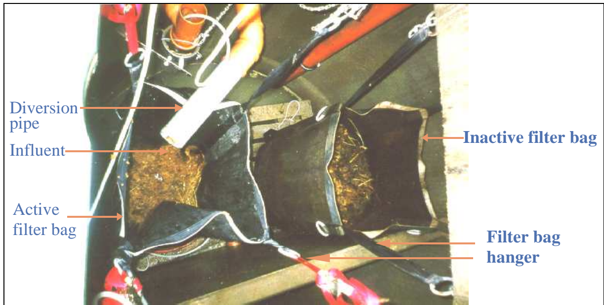
Figure 29: Rottebehälter with two filter bags in the pilot project Lambertsmuehle
