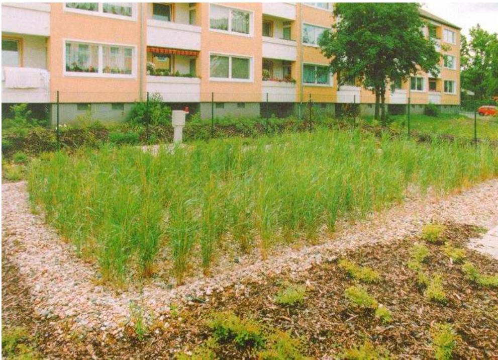
Figure 2: Unsaturated vertical flow constructed wetlands in Hannover, Germany
