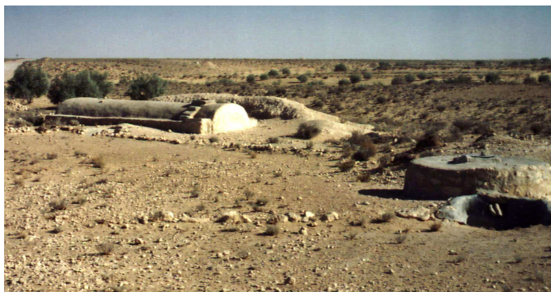
Figure 19: Fsaoui (left) and majel (right) with a natural impluvium (Photo: Meinzinger)
