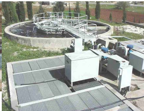
Photo 4: Wastewater treatment plant/ contact stabilization system/ Birzeit University
