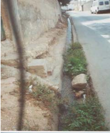
Photo 1: Wastewater disposal in open channels/ Al-Jalazoun Palestinian Refugee Camp/ the West Bank/ Palestine (Mahmoud et al., Submitted)
