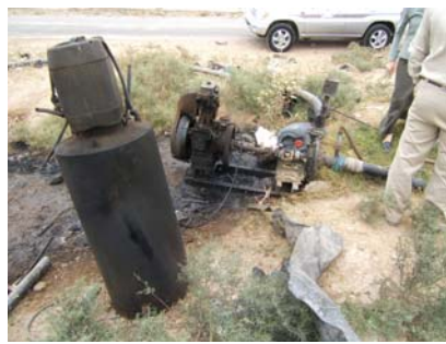
Figure 2: Diesel powered centrifugal pump – no filter
