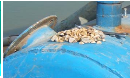
Figure 5: Oversized media used in the Traditional Sand Filter
