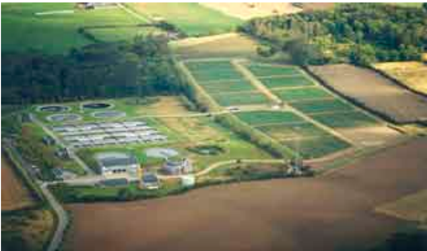
Figure 4: Kolding Sludge Reed Bed System (Denmark)
