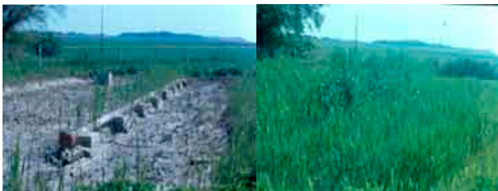
Figure 7: 1 st stage filter 3 and 10 weeks after sludge withdrawal, french plant (Liénard, 2003)
