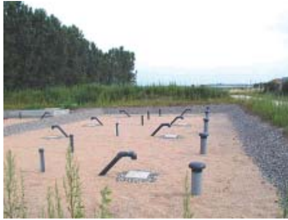
Fig. 6: 1 st STAGE BED AFTER COMPLETION AND BEFORE REED PLANTING
