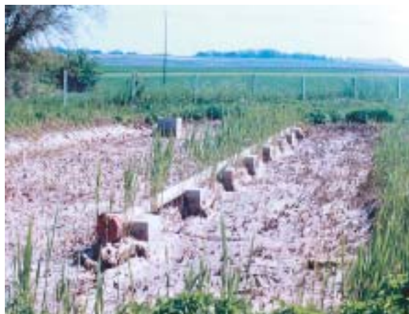
Fig. 7: 1 st STAGE FILTER THREE AND 10 WEEKS AFTER SLUDGE WITHDRAWAL, FRENCH PLANT
