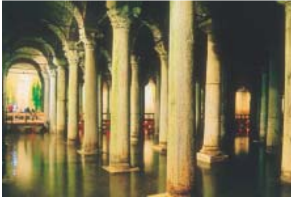
Fig. 2: YEREBATAN CISTERN IN ISTANBUL
