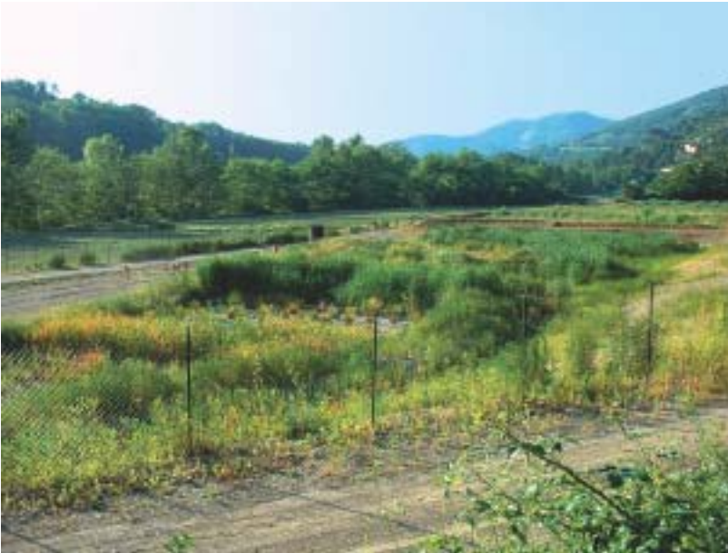
Fig. 1: A 6.000 m 2 COMBINED CW FOR THE TREAT- MENT OF WASTE- WATER OF A 3.500 INHABITANTS COMMUNITY
