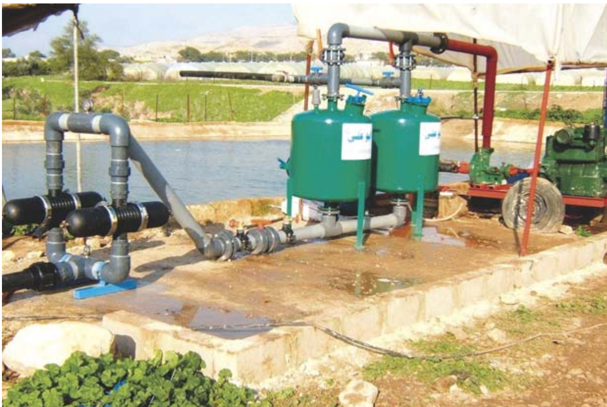
Fig. 4: IMPROVED DOUBLE-TANK FILTER IN A PILOT FARM (MREA DESIGN)
