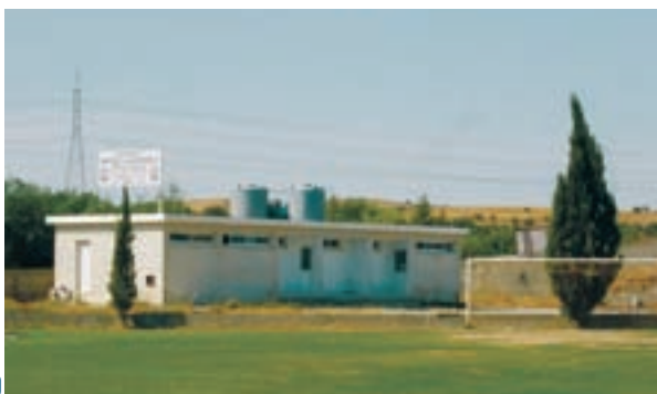
Fig. 5 GREY WATER TREATMENT PLANT AT A FOOTBALL FIELD
