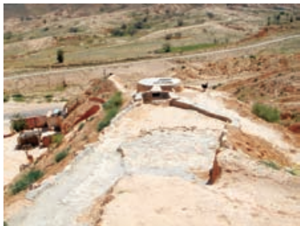
Fig. 6 RURAL RAIN WATER CISTERN, MATMATA
