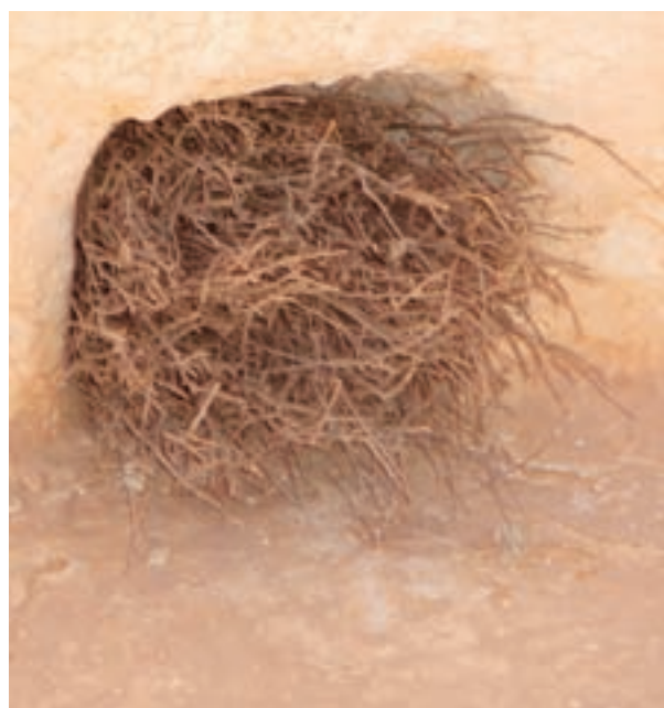
Fig. 4 AS TRADITIONAL FILTER HARD DRY THORNY PLANTS WORK FOR PROTEC- TION OF CISTERN AGAINST RODENT AND WASTE
