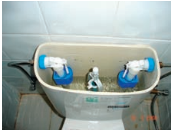
Figure 2 DUAL, NETWORK (GREYwater RECYCLING / POTABLE WATER) FOR TOILET FLUSHING (POTABLE WATER VALVE BEING ALWAYS CLOSED)
