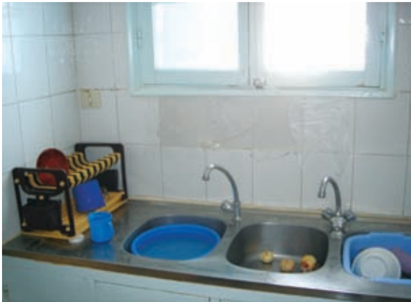
Fig. 10 THE KITCHEN IS CONNECTED TO RAINWATER (LEFT FAUCET) AND PUBLIC MAINS (RIGHT FAUCET)
