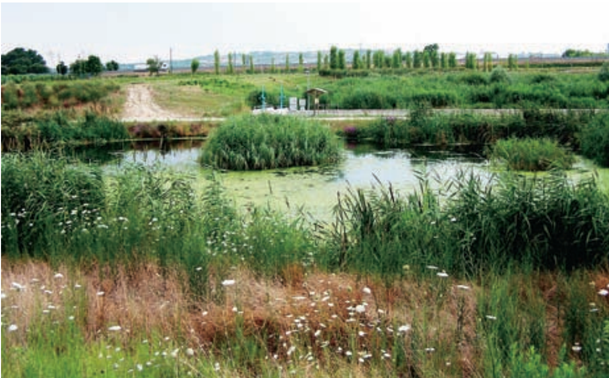
Fig. 3 HYBRID CONSTRUCTED WETLAND FOR ENHANCED DENITRIFICATION AT THE MUNICIPAL WASTEWATER TREATMENT PLANT IN JESI, ITALY
