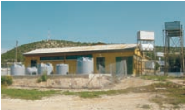
Fig. 4 GREY WATER TREATMENT PLANT AT AN ARMY CAMP
