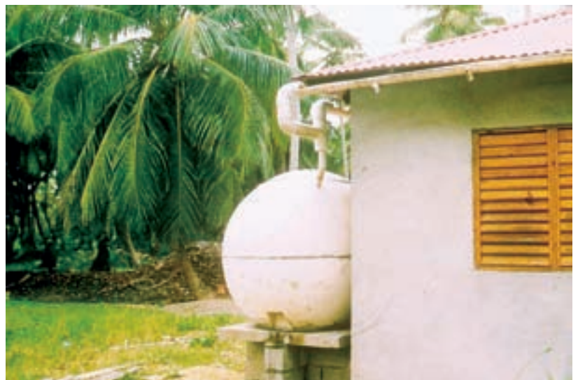
Fig. 3 IN THE DOMINICAN REPUBLIC RAIN WATER SUBSTITUTES DRINKING WATER AND IS DIRECTLY LED TO THE KITCHEN WITHOUT THE HELP OF A PUMP
