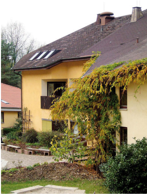
Fig. 13: ►► HAUS TOBIAS: LAUNDRY WASHED WITH RAINWATER
