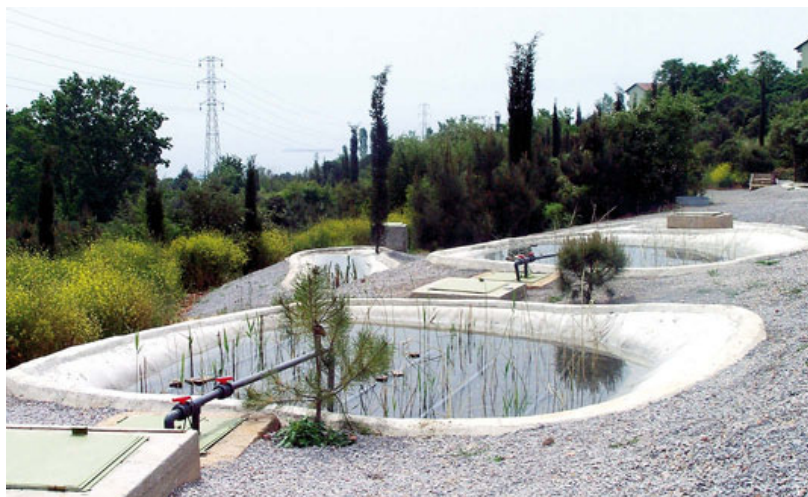
Fig. 3: CONSTRUCTED WETLANDS FOR BLACKWATER TREATMENT (VERTICAL FLOW, RECENTLY PLANTED)
