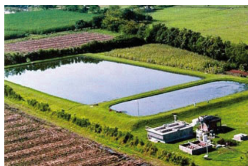
Fig. 4: WASTEWATER TREATMENT AND RESTRICTED IRRIGATION IN VALLE DEL CAUCA, SOUTHWEST COLOMBIA: THE WASTEWATER FROM THE SMALL TOWN OF GINEBRA IS TREATED IN AN ANAEROBIC POND AND A SECONDARY FACULTATIVE POND AND THE EFFLUENT USED TO IRRIGATE SUGAR CANE
