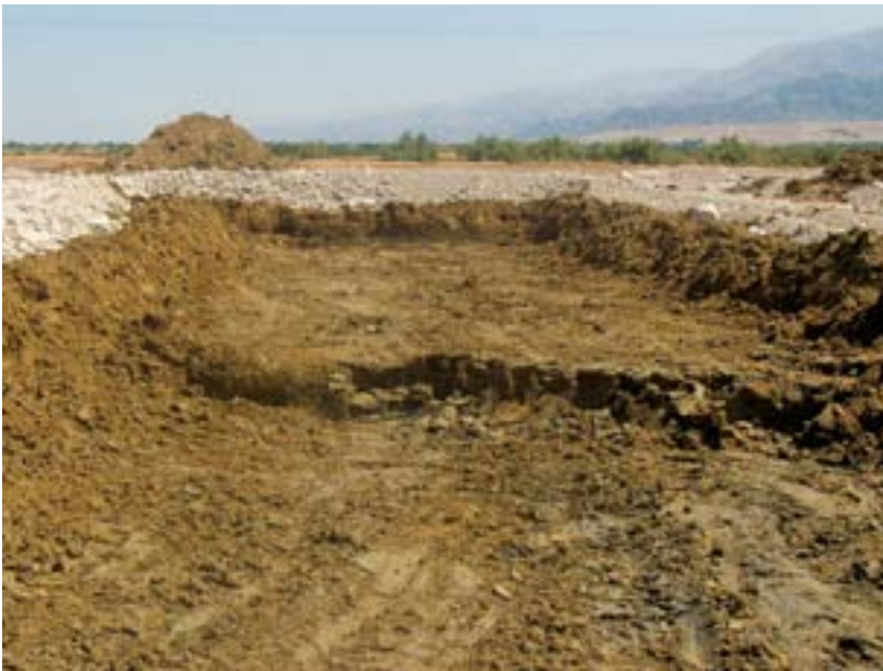
▲ Fig. 2: EXCAVATION OF EARTH
