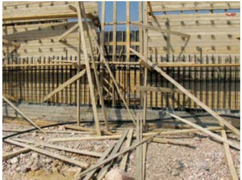
▲ Fig. 5: FORMWORK
