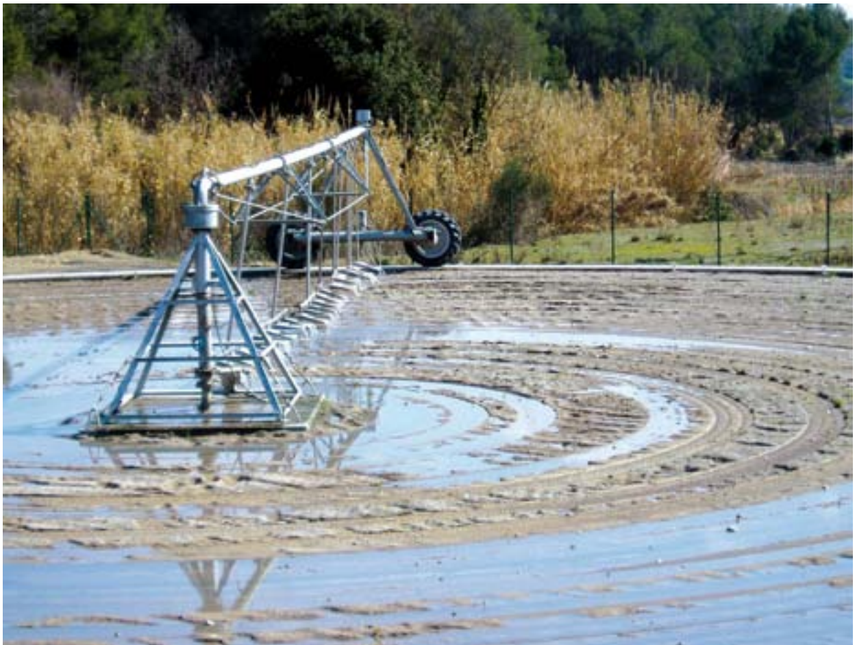
► Fig. 2: OVERLOADED INFILTRATION PERCOLATION PLANT
