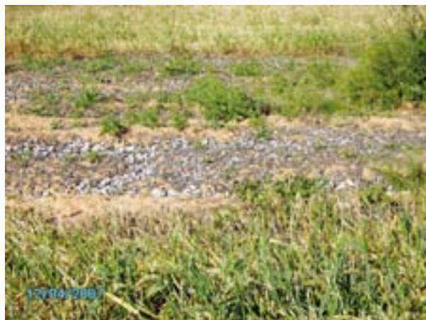
▲ Fig. 2: MARKS OF TREATED WASTEWATER ON THE SOIL
