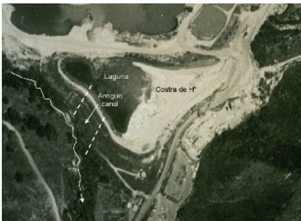
FIGURA 5. Vista aérea de la presa de Tapo Canyon previa a su rotura (Foto de Northridge Collection, Earthquake Engineering Research Center, University of California, Berkeley).
