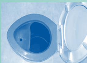
Photo: Self-made cement urine diverting toilet used in rural areas of Eastern Europe is hygienic and prevents groundwater pollution
