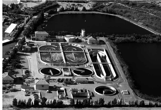
Figure 2 | Alhama: tertiary treatment plant.
