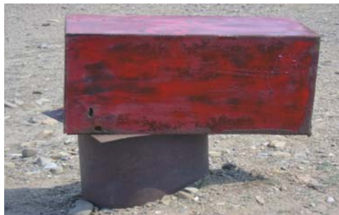
Fig. 16. Installed instrument for groundwater monitoring.
