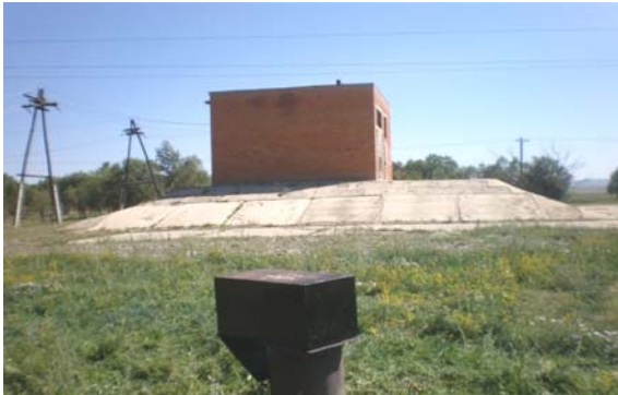
Fig. 9. Monitoring point 1 near the well 8.
