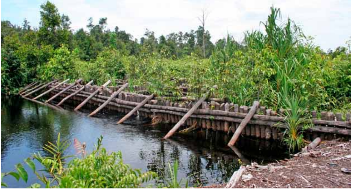
Dam built by Wetlands International in channel at Mentangai, Central Kalimantan, Indonesia Photo: Marcel Silvius
