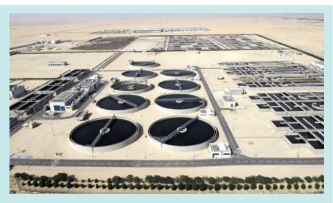
secondary treated water from the biological treatment system is then directed to the reclamation plant.
