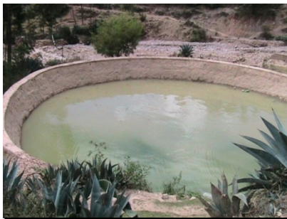
Small dam to catch water
