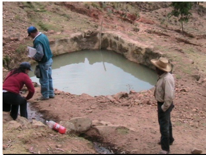
Rudimentary reservoir of water
