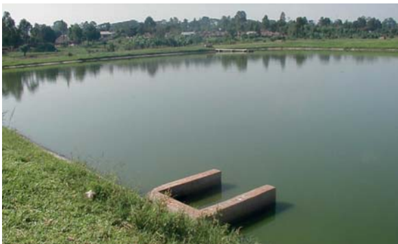
Waste Stabilization Pond in Gulu, Uganda
