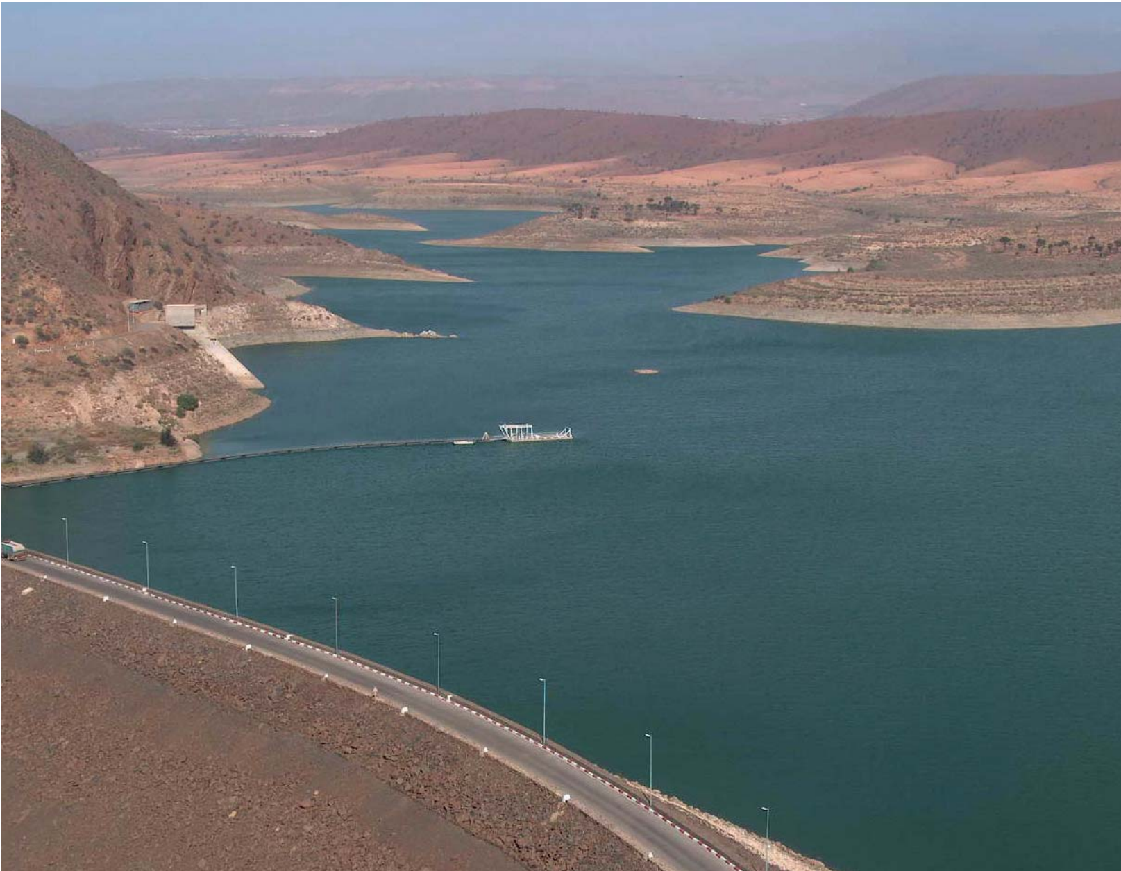
Youssef Ben Tachfine Dam, Morocco
