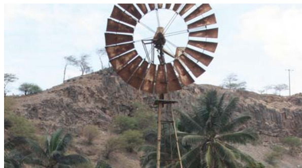
Windmill water pumping, Cape Verde
