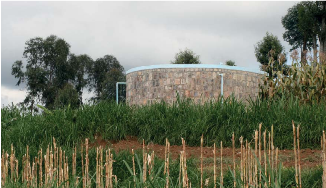
Water Reservoir, Rural Rwanda
