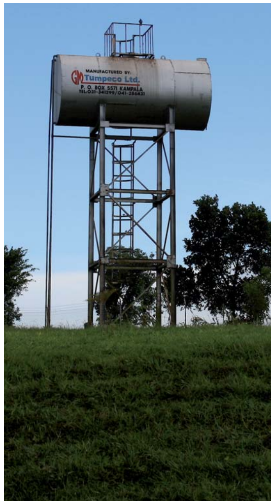
Water Storage Tank, Uganda
