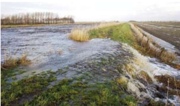
Figure 23 Overtopping of an unprotected river dike (Sicherer Deich, 2008)
