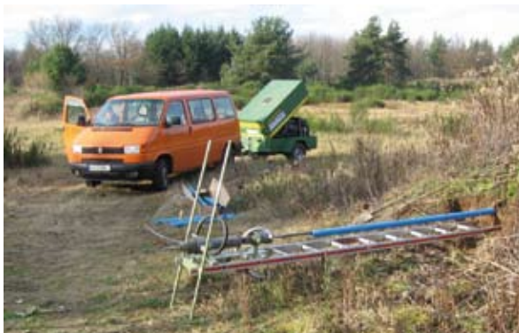
Figure 28 Installation of a drainage element in the dike body (Draenelemente, 2008)
