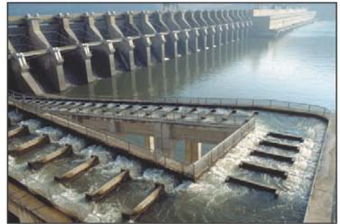
Fish ladder and spillway at John Day Dam (WA)
