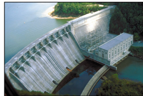
Allatoona seasonal storage project (GA)
