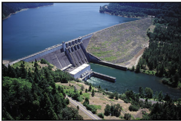
Lookout Point Dam (OR)
