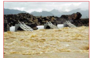
Tillamook flooding with advance measures in place.
