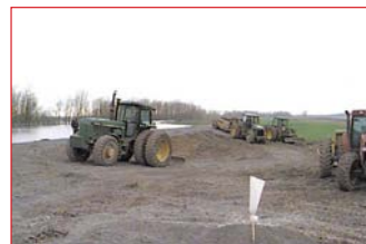
Emergency repair work on existing levee in Midwest.
