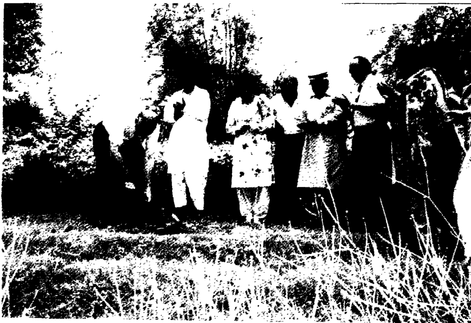
Figure 4-2. Ground breaking ceremony for the Department of Women's Studies building
