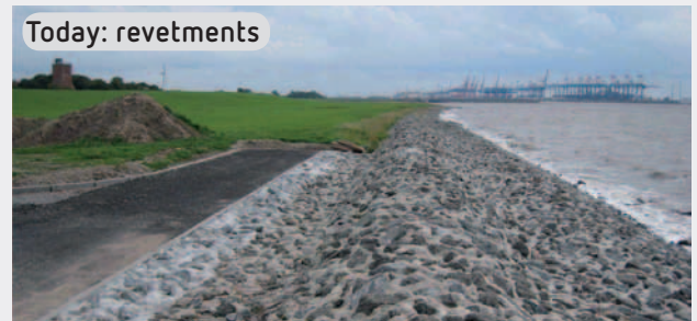
Figure 13. Development of artificial embankments which lead to a loss of natural habitat. Credit: Andreas Tesch (bottom).
